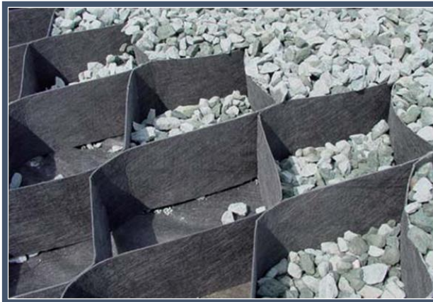
Figure 9 Examples of Cellweb filling with angular stone
